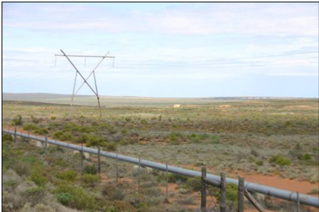
Figure 6: Power line infrastructure traversing the study area.
