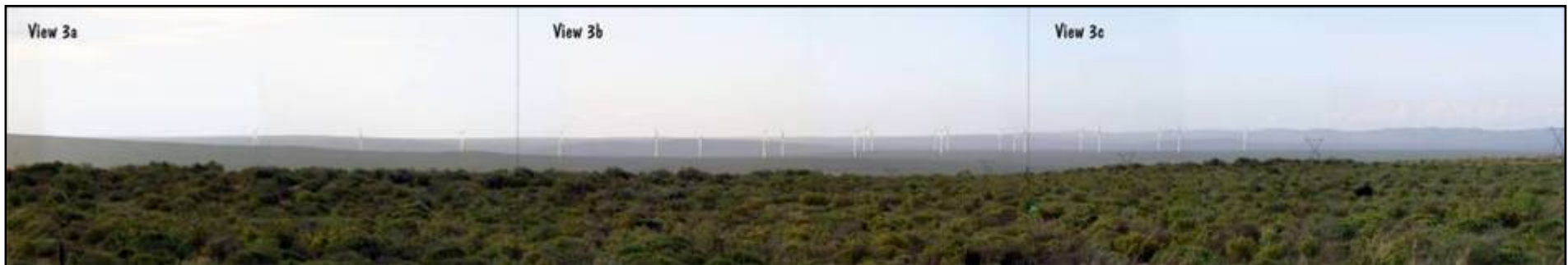
Figure 10b: Post-construction panoramic overview from Viewpoint 3 (indicating enlarged photograph sections).
