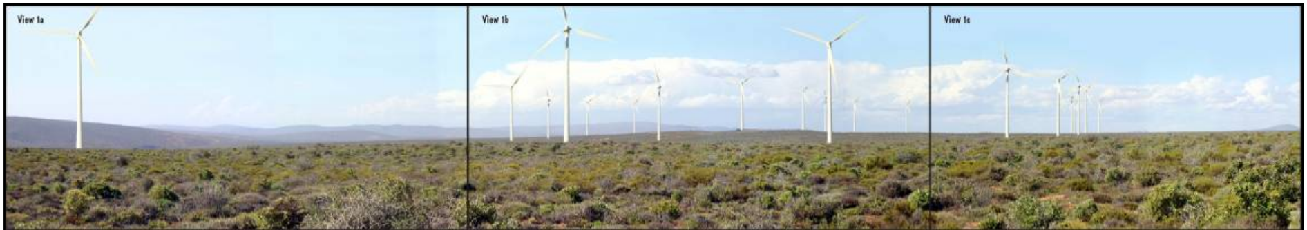
Figure 8b: Post-construction panoramic overview from Viewpoint 1 (indicating enlarged photograph sections).
