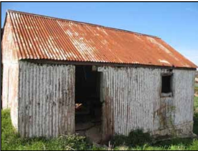
Figure 66: The corrugated iron structure with bricked in walls.
