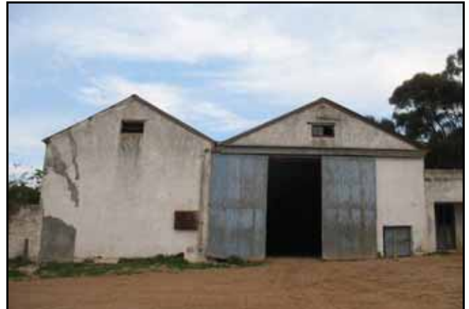
Figure 34: The north end of the barn.
