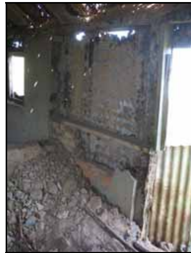
Figure 67: View of the inside of the ruined corrugated iron structure.
