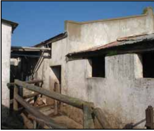
Figure 49: The core of the dairy with its thick wall revealed in a Doorway and the northern addition with thinner walls.
