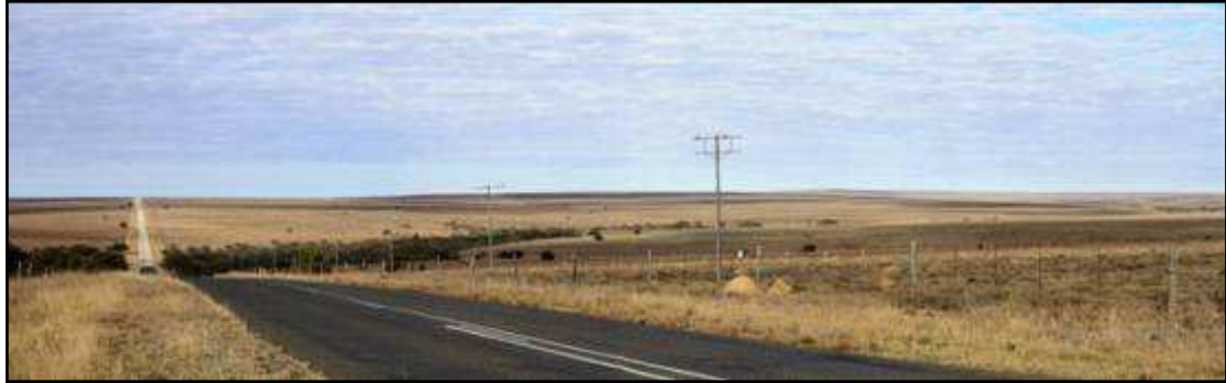
Figure 9a: Pre-construction panoramic overview from Viewpoint 2.
