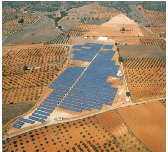
Figure 1: An example of a 20MW PV solar facility
