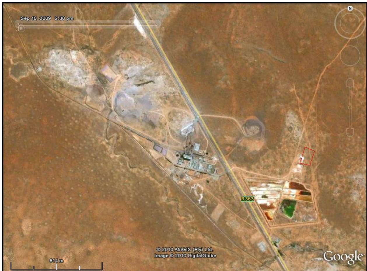
Figure 10: Aerial view of the area showing the existing mining facilities, spoil heaps, slimes dams and the landfill site.
