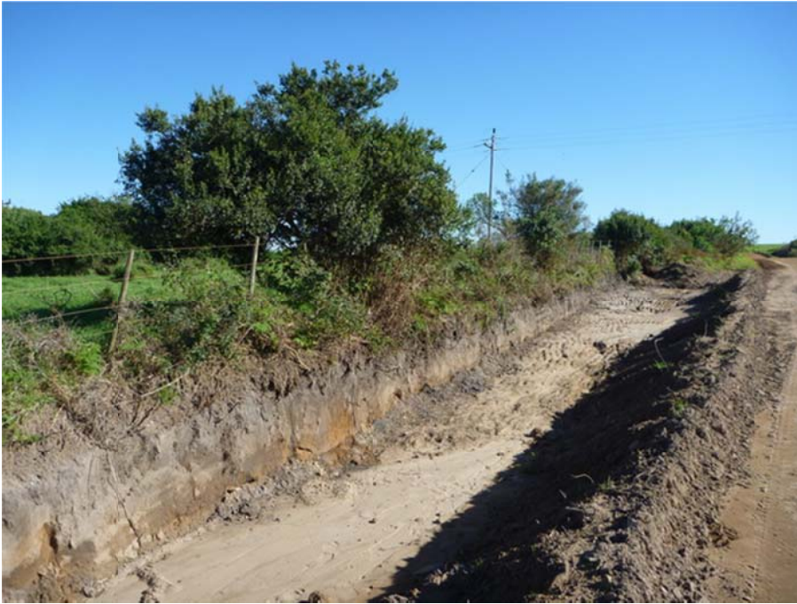
Figure 9 Fresh road cutting on the southern edge of the site
