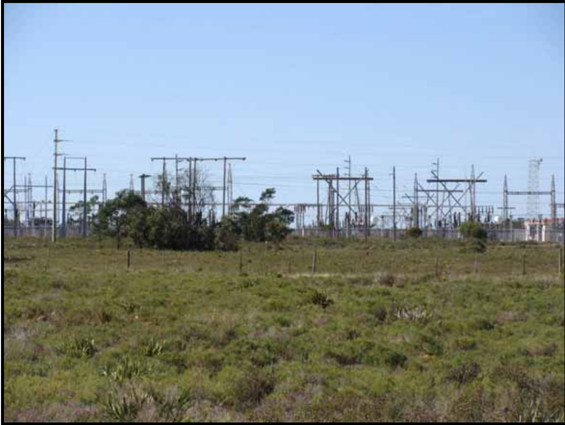
Photograph 1.2: Existing Melkhout substation located north of the N2 National Road
