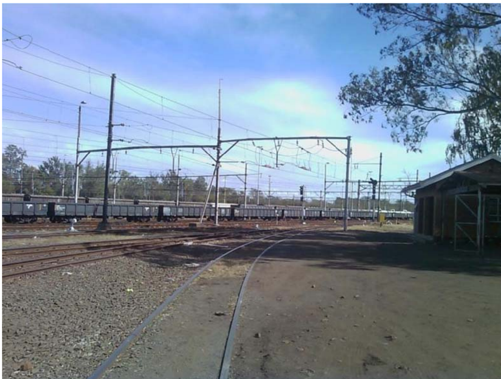
Figure 5: General view – Komatipoort Railway Station
