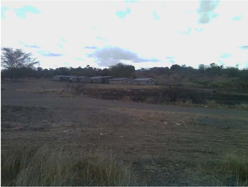
Figure 9: Komatipoort Railway Station - Residential area built next to the west yard
