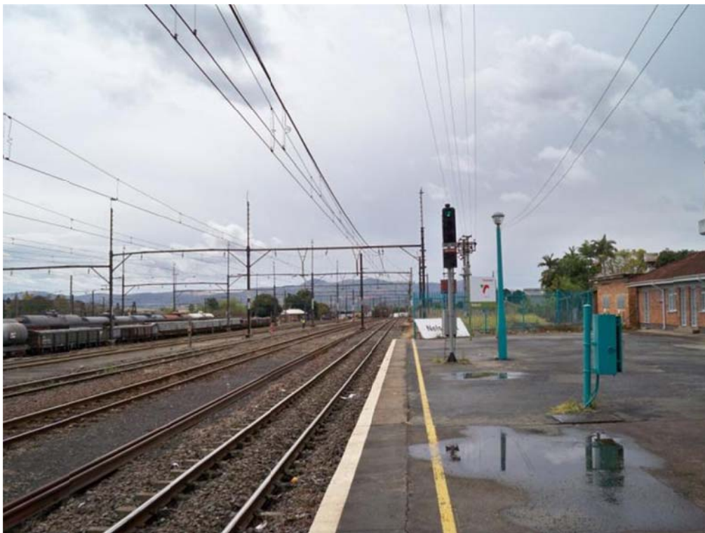
Figure 1: Nelspruit Railway Station – General view
