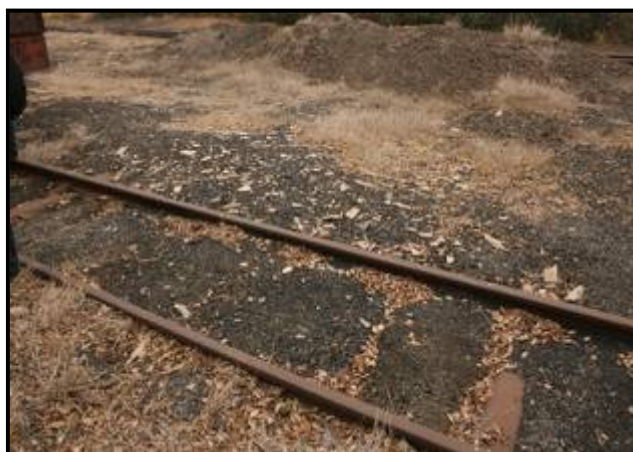
Figure 7: Komatipoort – Mixed Asbestos Waste
