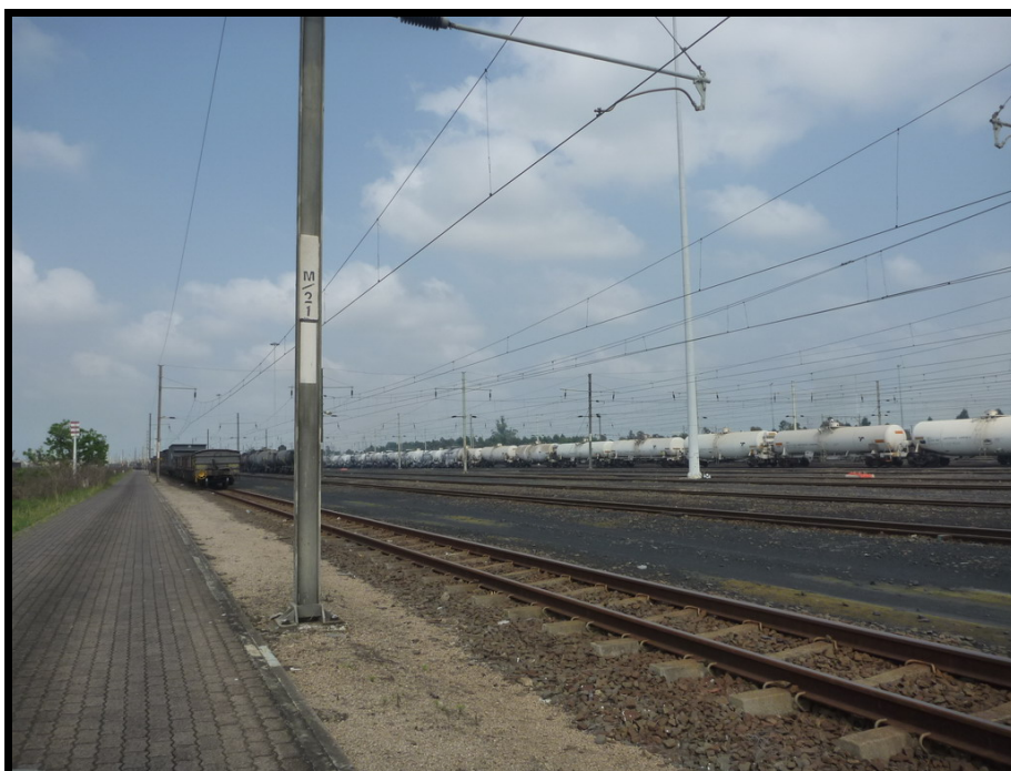
Figure 17: Photo indicating the transformation of the naturally occurring soils owing to development on the Nsese yard
