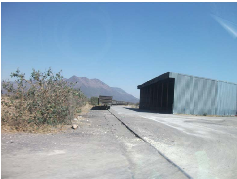
Figure 4: Apiesdoring – SAMREC Factory utilising shed next to the Apiesdoring Station
