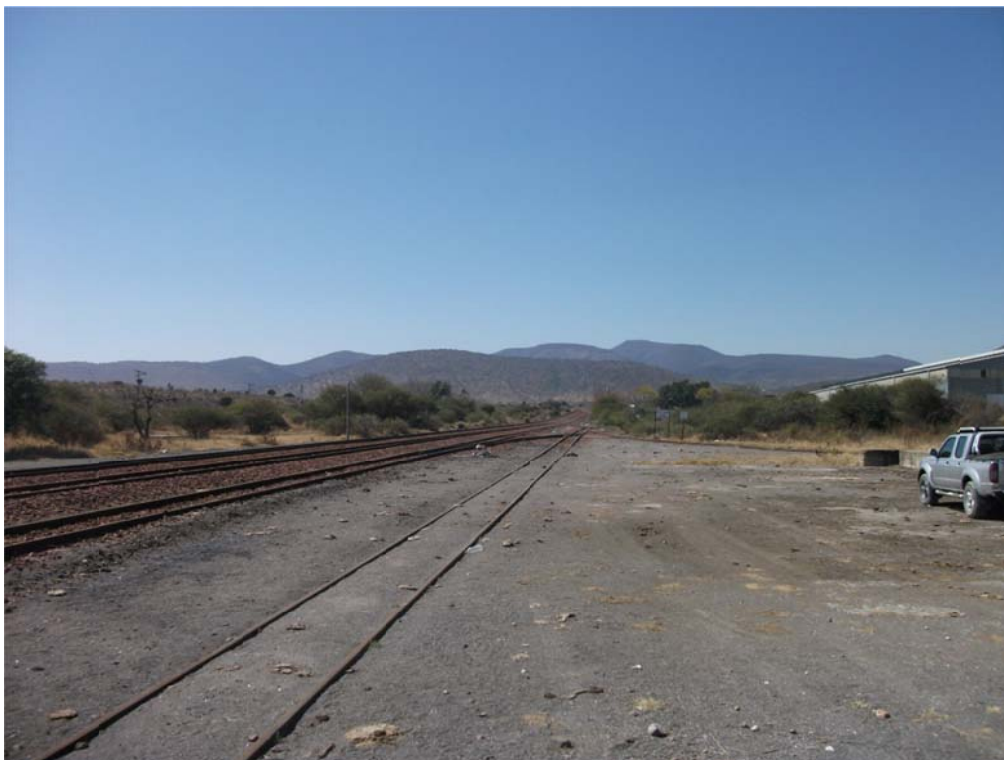
Figure 5: General view – Apiesdoring Railway Station
