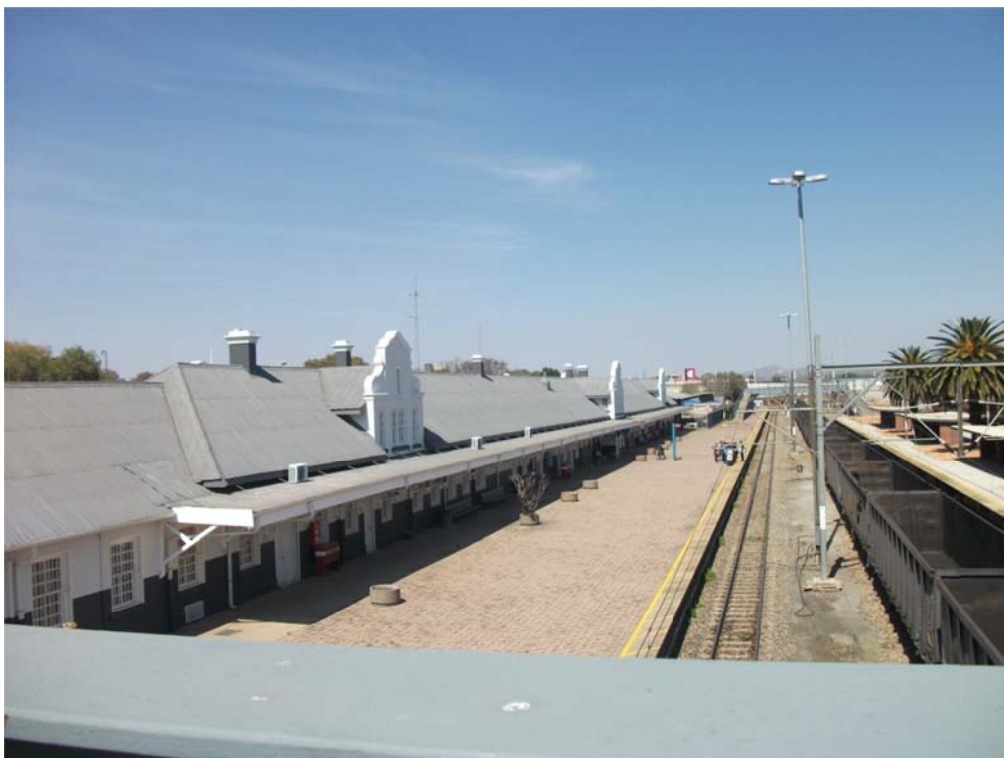
Figure 2: Polokwane Railway Station – General view
