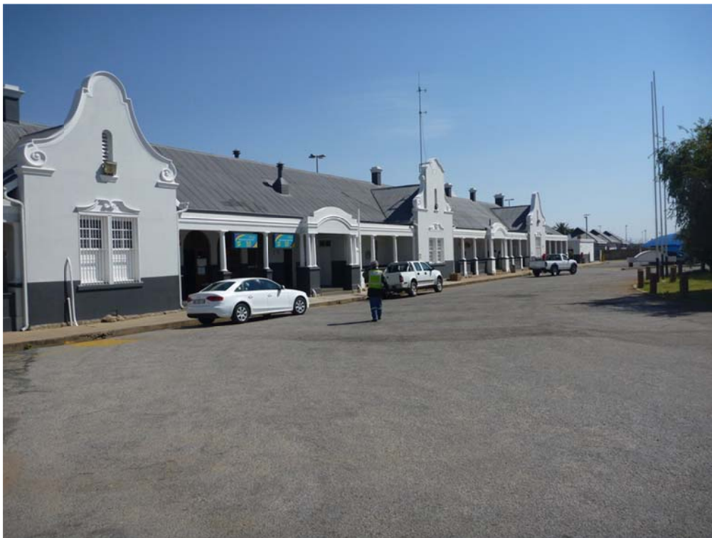
Figure 1: Polokwane Railway Station – General view
