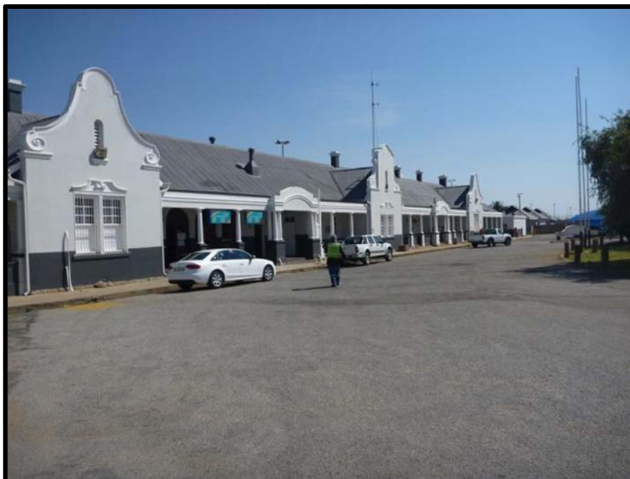
Figure 8 Photo illustrating the transformation of the natural occurring soils owing to development
