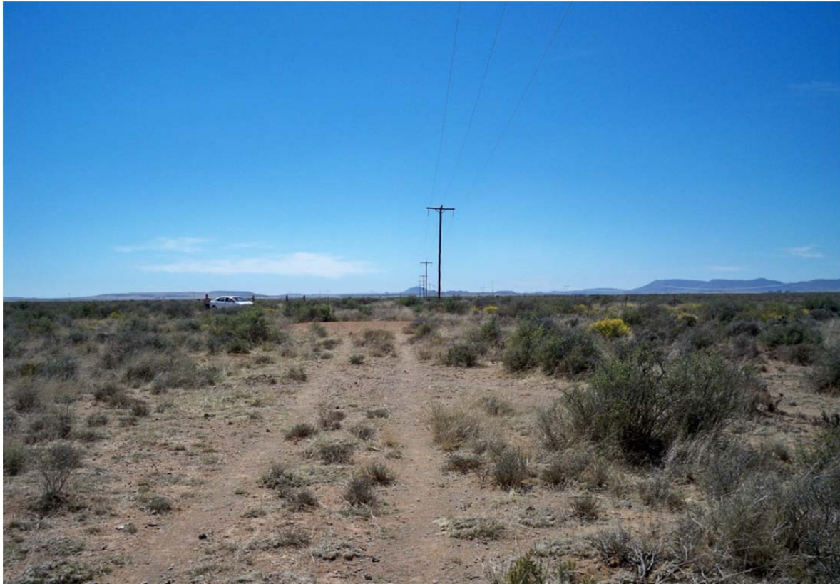
Figure 10: Some of the electrical infrastructure that crosses the site.
