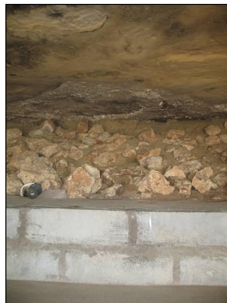
Figure 6: View of the interior of ON001. Photo: 02.06.2010.
