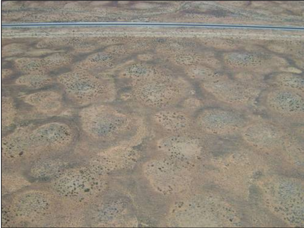
Figure 1: Aerial view of a section of the N17 national road, running between Aggeneys and Springbok.
