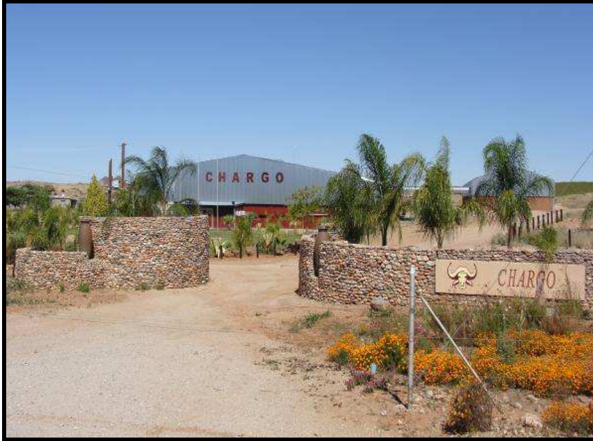
Photograph 2.7: Chargo packing facility
