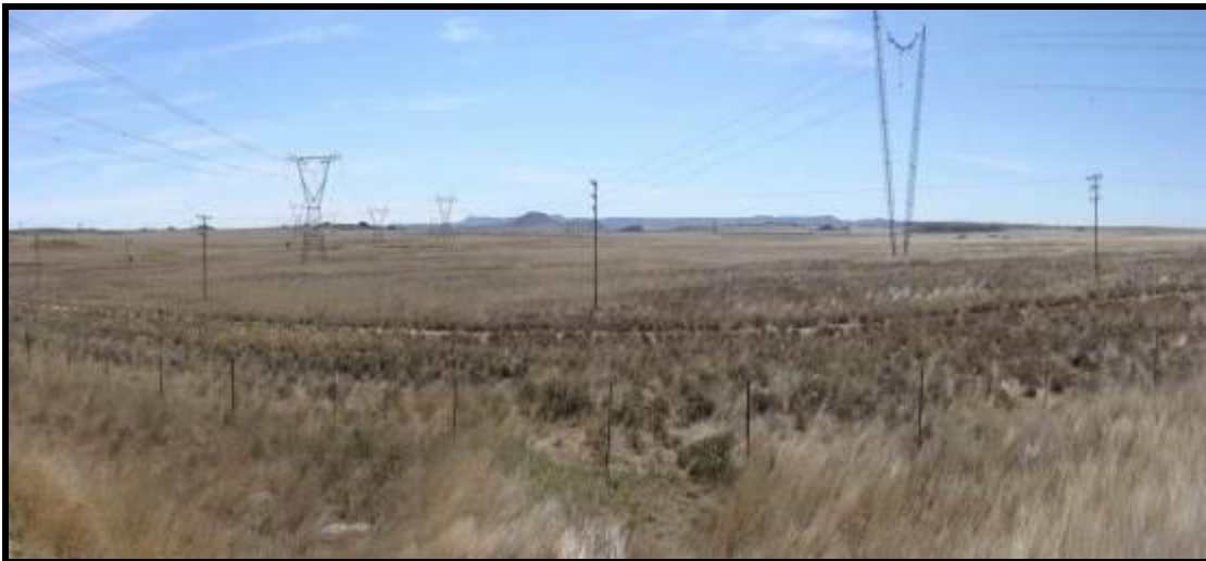
Photograph 2.3: View of existing power lines that traverse the site
