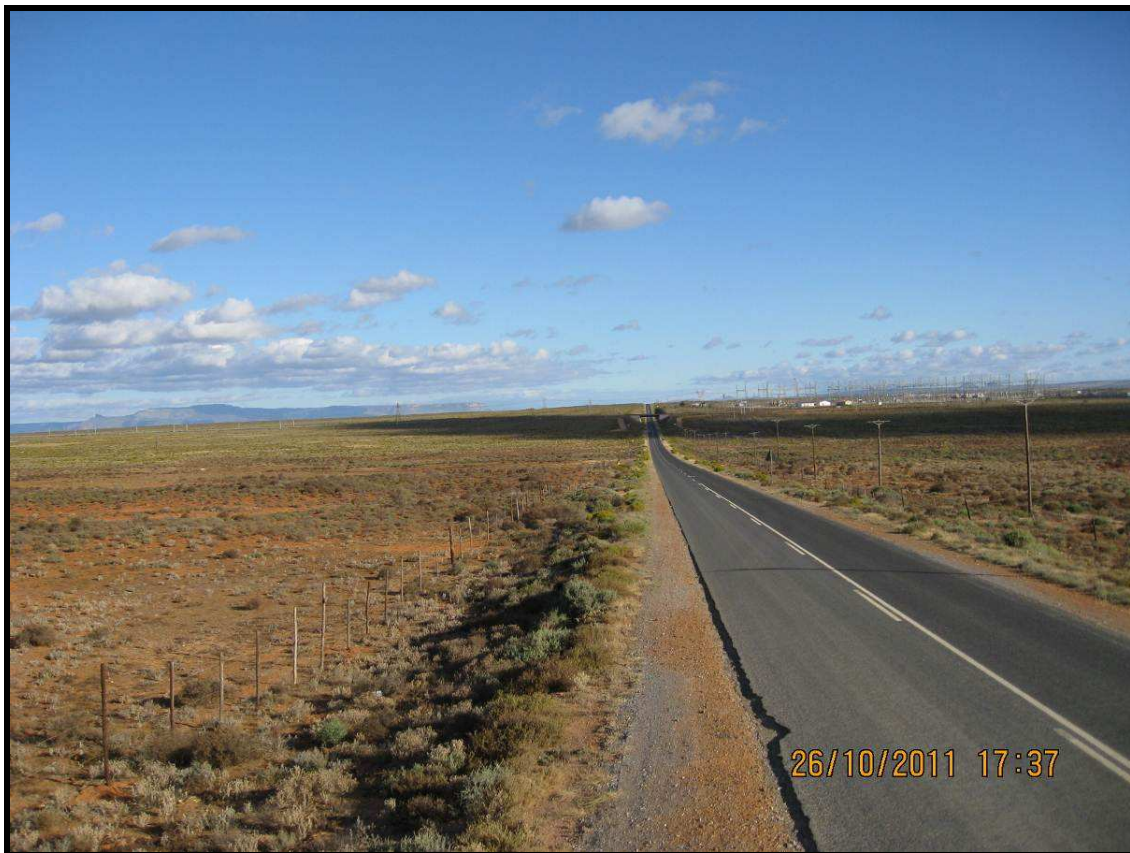
Photograph 3.2: R362 "Holrivier Road" - view from north-east – INCA site located on left far distance; Eskom Juno on the right
