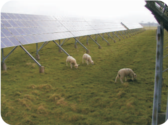
Figure 1: Photo showing view of photovoltaic panels from ground level (Picture source www.wikipedia.com )
