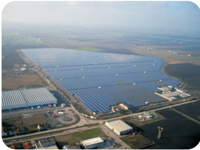
Figure 2: Photo showing aerial view of a PV facility (Picture source www.sunedison.com )
