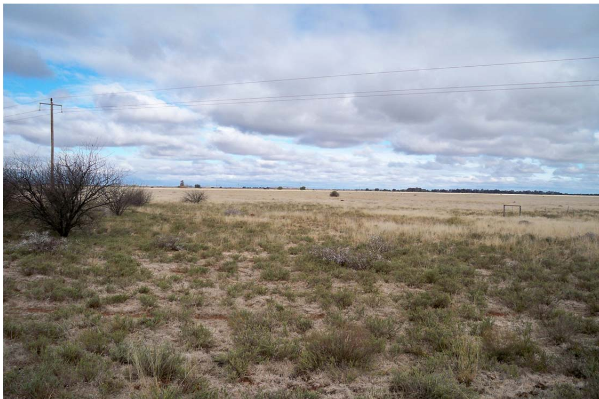
Figure 1: Photo showing some of the electrical infrastructure that crosses.
