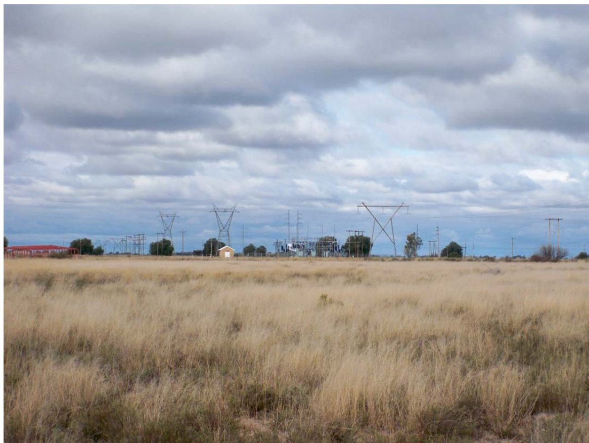
Figure 6: View of Ritchie substation from the site.
