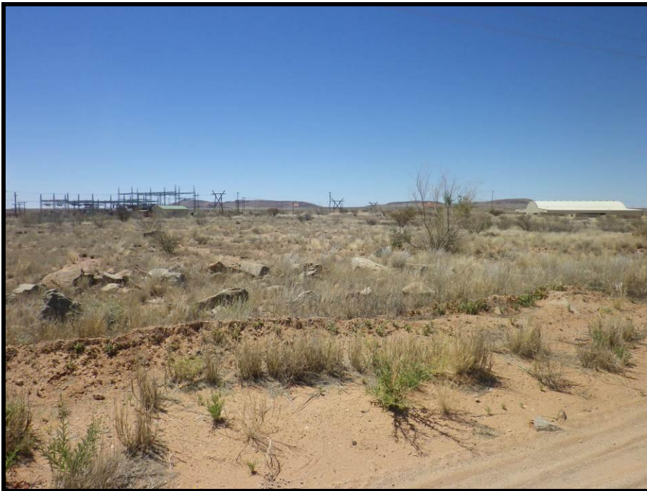
Photograph 3.4: View of Oasis substation and Orange River Winery ~ 2 km north east of Keimoes
