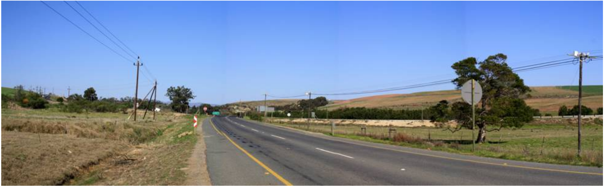
Figure 7a: Pre-construction panoramic overview from Viewpoint 3, looking at the Klipheuwel portion of the proposed WEF facility.
